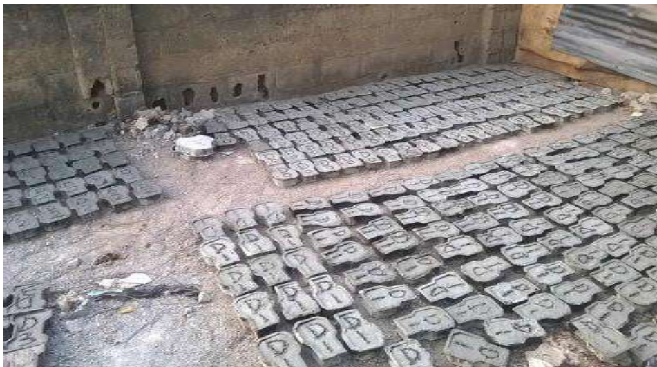
Figure 13: CSA Interlocking Paving Stones
