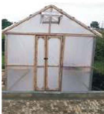
Plate 7: Constructed solar tent dryer
