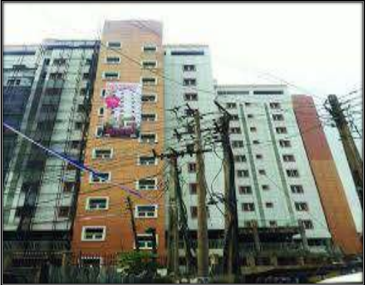
Plate 9: Newly Redeveloped High-rise Condominium (Jelili, et al , 2020)
